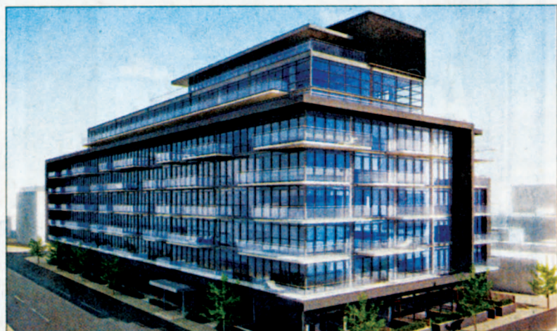
The nine-storey building planned for Broadview Ave., just north of Queen St. E., is called Leslieville Lofts, even though it's not in Leslieville.
