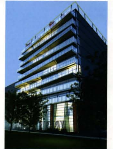
Parc Lofts – the latest addition to LDC’s portfolio, is an intimate loft building backing onto a park in the heart of King West.
